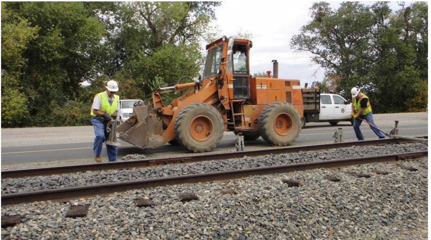
Hop-scotching down the line. As the tamper tamps up the raised sections, the jacks are loaded into the bucket of the loader which then heads south. Clem takes a jack for placement as Ed continues to lift-up the west rail level with the east
